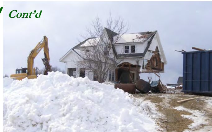
Left - demolition of farmhouse with excavator
