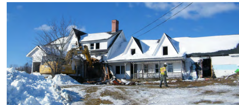
Lowery Farmhouse on Demolition Day February 24, 2014
