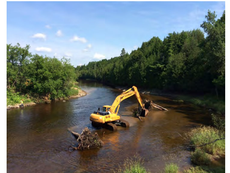
Log cluster being installed north of Lowery Bridge
