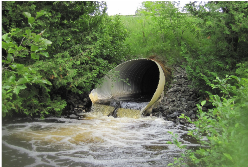
Bithier Brook, 2014. Example of hanging culvert impeding fish passage and impacting aquatic connectivity. Photo courtesy MDEP.
