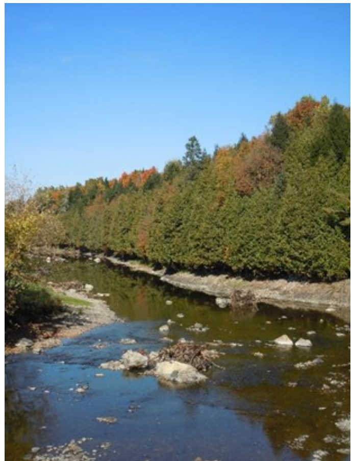
Placement of logs and boulders in the Meduxnekeag River
