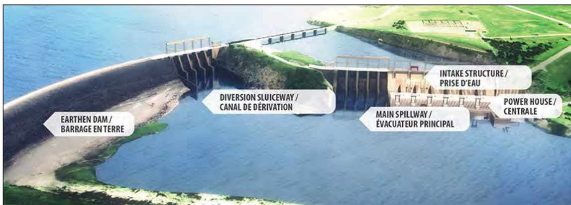
Figure 3-10. Schematic Representation of the Existing Mactaquac Dam
