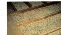
Vermiculite insulation between attic joists
