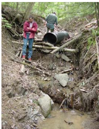
Drainage ditch and erosion damage behind Millar Civic Center in Houlton
