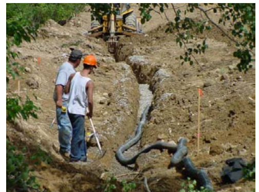
Newly installed perforated underdrain
