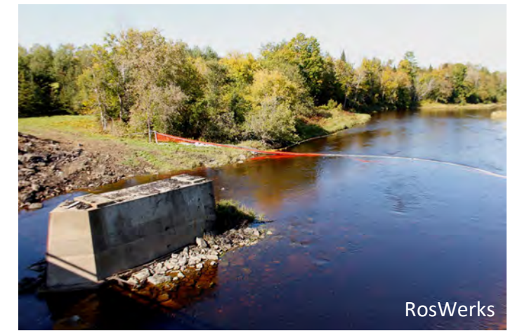
DOT dam removal September 20, 2021. Note boom to catch debris in photo above right.
