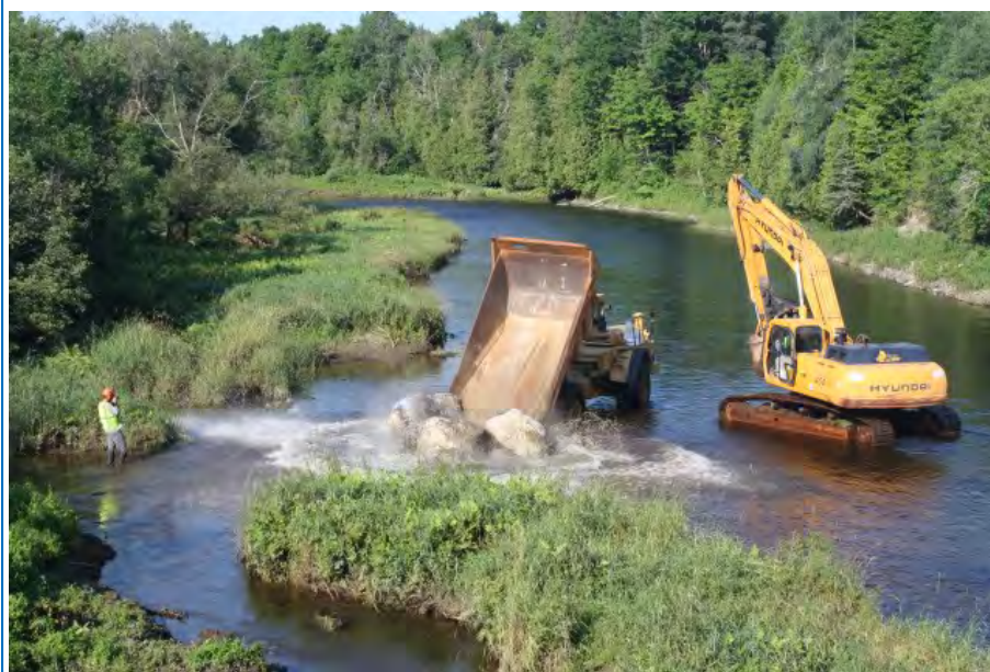
Figure 5. Habitat Improvement Project. Boulders are placed in the Meduxnekeag River to create a more natural aquatic habit for fish. Photo credit: USFWS . https://usfwsnortheast.wordpress.com/2014/09/05/wabanaki-days-in-maine/
